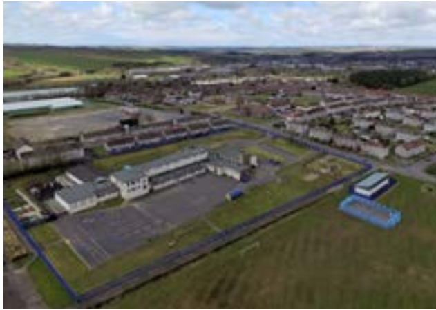
Aerial View from South East
